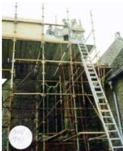
Repairs in progress, November 1991
