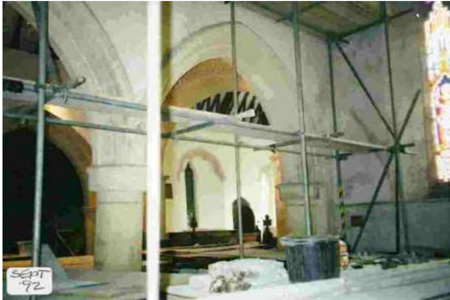
Internal repairs, September 1992
